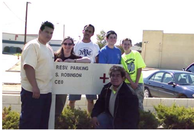
YouthBuild students and instructor Chris Hammond (3 rd from left) install sign for Sue Robinson (2 nd from left)
